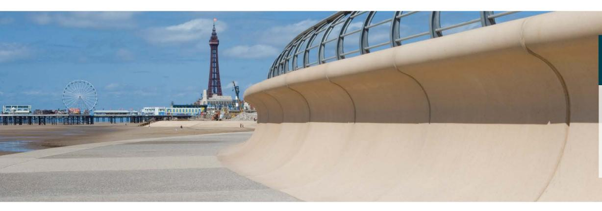
Regen provides a superior, lighter-coloured finish than concrete made using Portland cement-only mixes.
