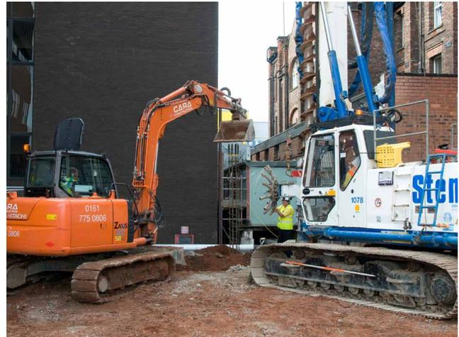
product from **Hanson Concrete** that has been developed with **Sika® Limited**, incorporating the admixture system **Sika® PilePak**, and has been specially formulated for CFA piling concrete to improve cage placement in dry and dense ground conditions. It gives improved cohesion properties and pumpability as well as reducing water loss, segregation and bleeding from the concrete.
