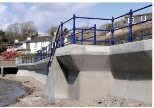
chloride attack and **Sika® Control 40** to reduce the potential for shrinkage. Expansion joints along the walkway were sealed with **Sikaflex®-AT Construction** multi-function joint sealant..
