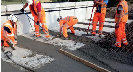
25N/mm² of strength within 24 hours in order to meet the exacting timescales for the project. Hanson's technical team designed a FastTrack mix which far exceeded this, initially hardening in 37 minutes and showing a strength gain of 40.5N/mm² in 24 hours.
