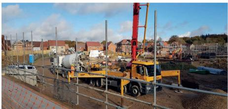
Council has used a self-compacting concrete mix so the testing regime required to confirm compliance was rigorous. Hanson provided a team of technicians at its Southampton batching plant to test the loads according to various British Standards to confirm that the requirements for appearance, flowability, viscosity, passing ability and segregation were met. As well as the testing at the plant, Hanson provided technical representation on site to ensure full support.
