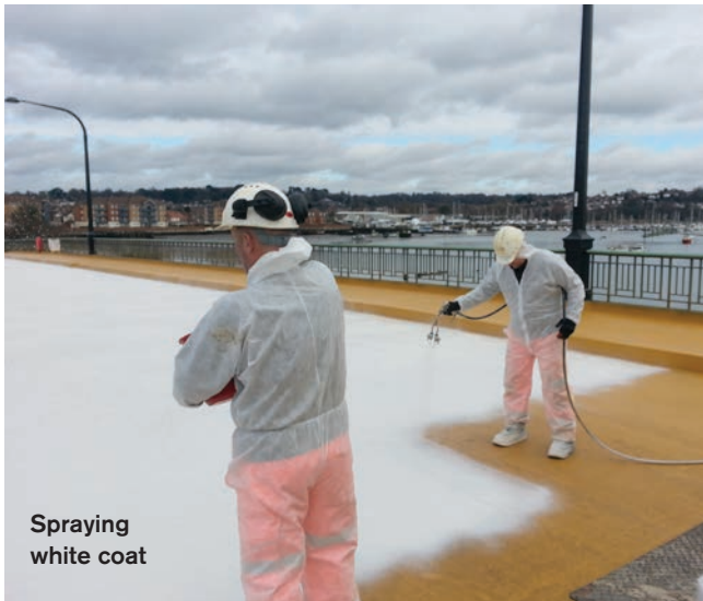
Spraying tack coat
