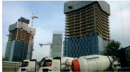
concrete containing 70 per cent Regen GGBS to minimise the production of heat and reduce the risk of thermal cracking.
